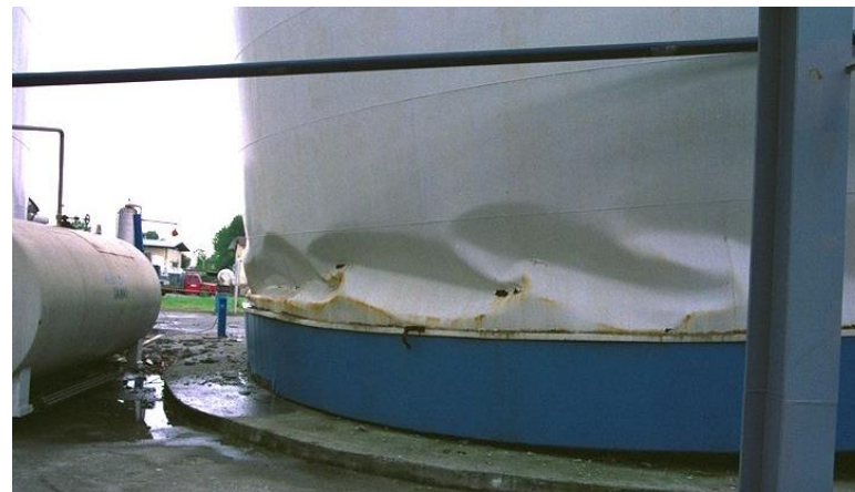
ELASTIC BUCKLING (Diamond shape)
