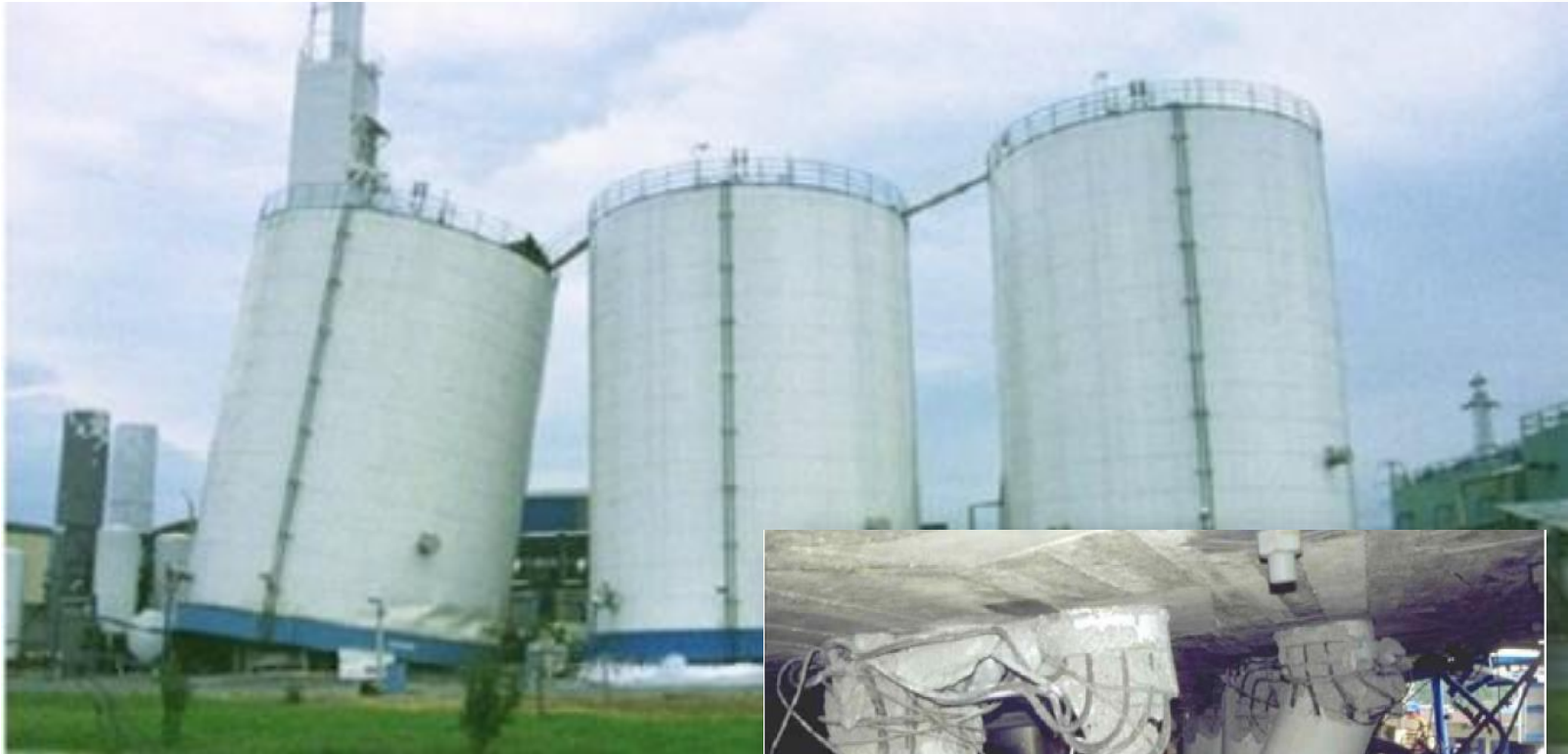
Storage tanks of Liquid Oxygen at Habas plant after the strong event of Itzmit (1999)
