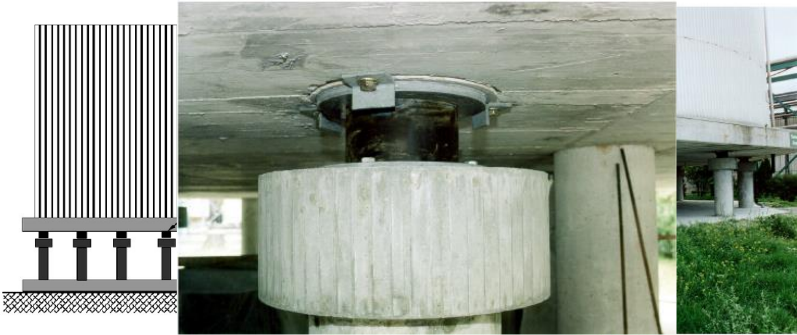
Seismic retrofitting of a steel tank using 26 HDRB isolators Switzerland
