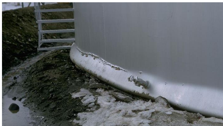
ELASTOPLASTIC BUCKLING (Elephant's Foot)
