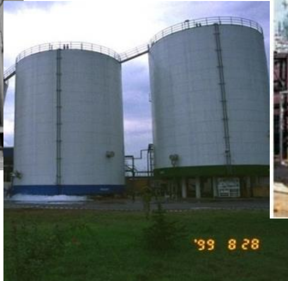
Cylindrical elevated tanks
