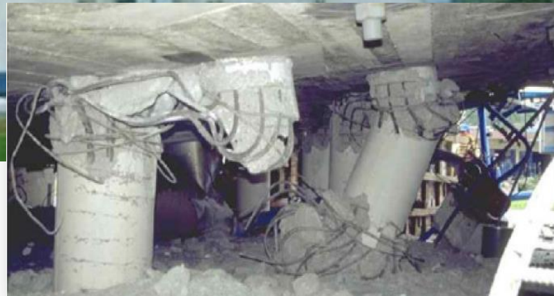
Storage tanks of Liquid Oxygen at Habas plant after the strong event of Itzmit (1999)
